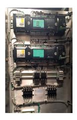
The BFM-II is ideally designed to upgrade existing substations with electro-mechanical relays and to provide real-time information and control over these highly reliable, yet limited, devices.
